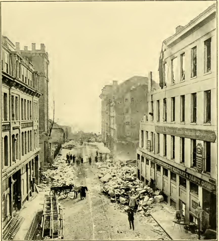
LOOKING DOWN SUMMER STREET, SHOWING RUINS OF SHIREVE, CRUMP, & LOW'S— HOVEY'S IN DISTANCE
